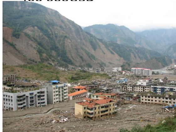
Photo: David Wald, USGS. Public domain https://www.usgs.gov/media/images/damage-2008-great-sichuan-earthquake-china
