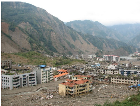
Photo: David Wald, USGS. Public domain https://www.usgs.gov/media/images/damage-2008-great-sichuan-earthquake-china
