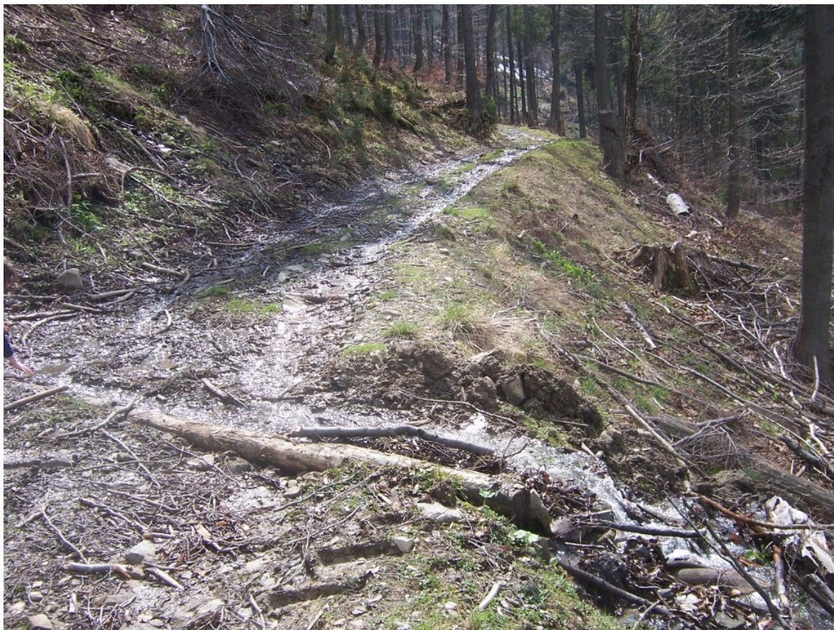
A waterbar on a forest road, the source zone of the Bystra stream
