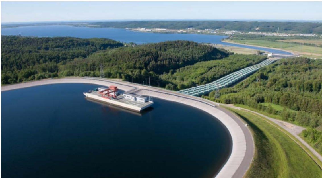
Fig 6: Pumped storage power plant in Żarnowiec, Poland
