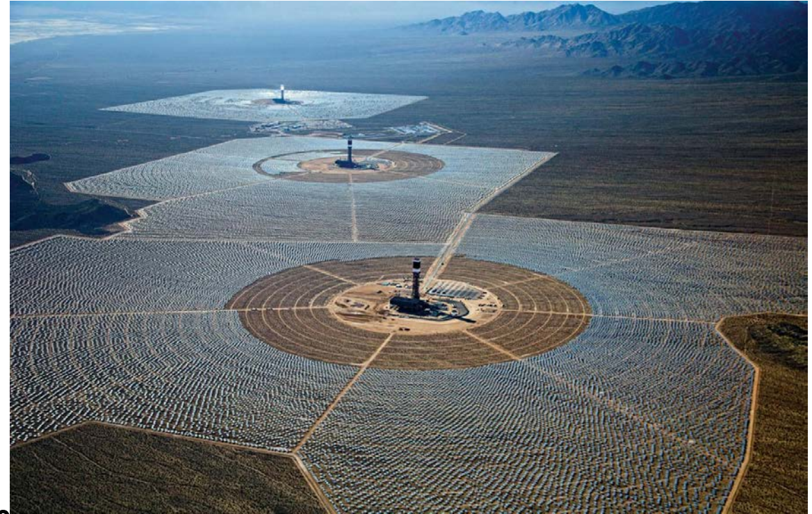
Fig 3: Solar thermal collector power plant, California
