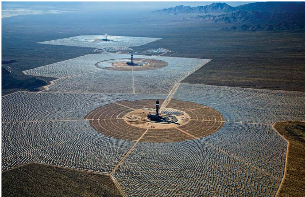
Fig 4: Solar Power Plant - Collectors, California
